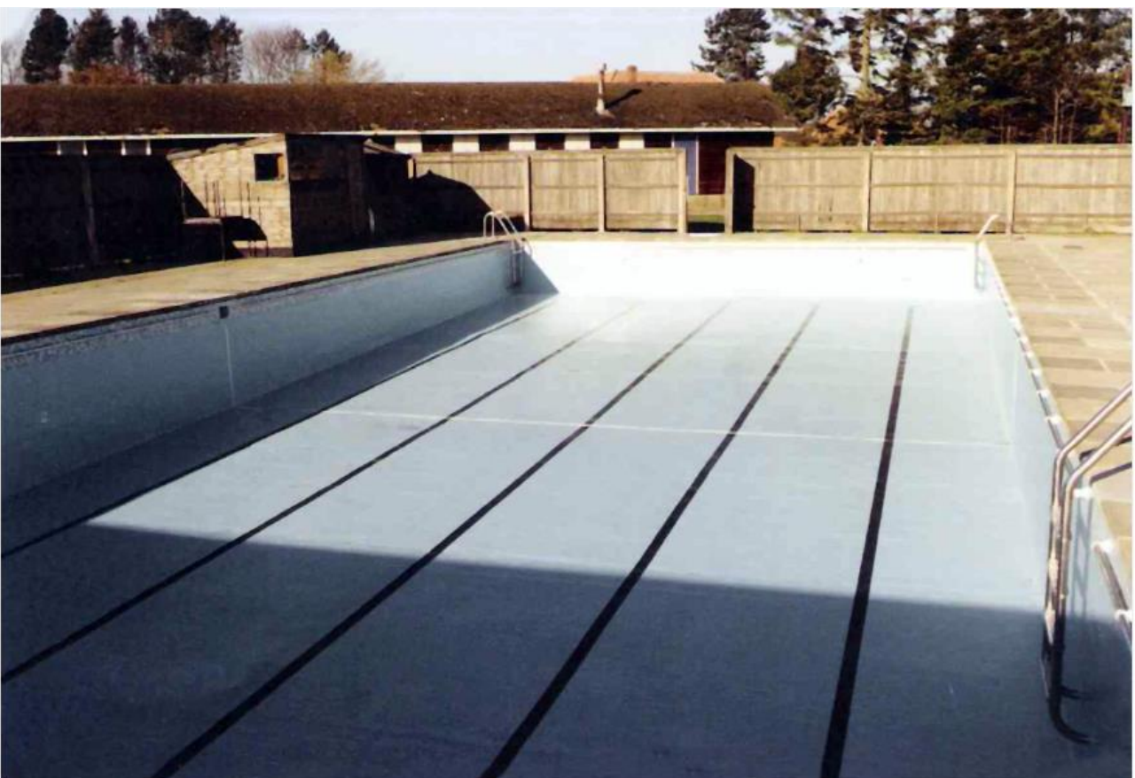
New Pool Lining 1987
