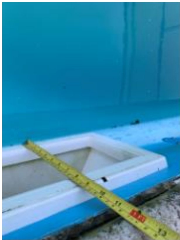
Photo 10: Site visit photos – Examples of the pools edge and weak junction of the coping stone and lining
