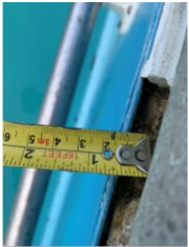
Photo 10: Site visit photos – Examples of the pools edge and weak junction of the coping stone and lining
